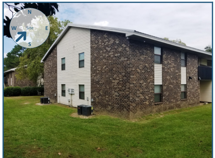
View of site from the southwest
